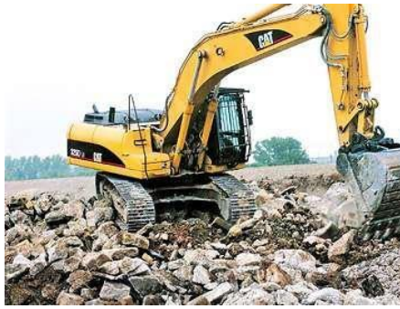
Fig. New Power Shovel
